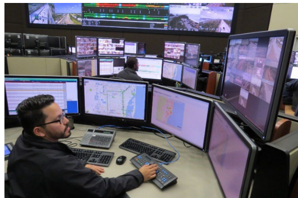
Traffic Management Center
