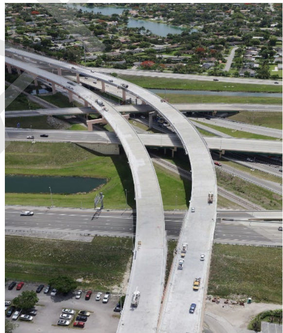
SR 874 Northbound/Southbound Connector Bridges to SR 874
