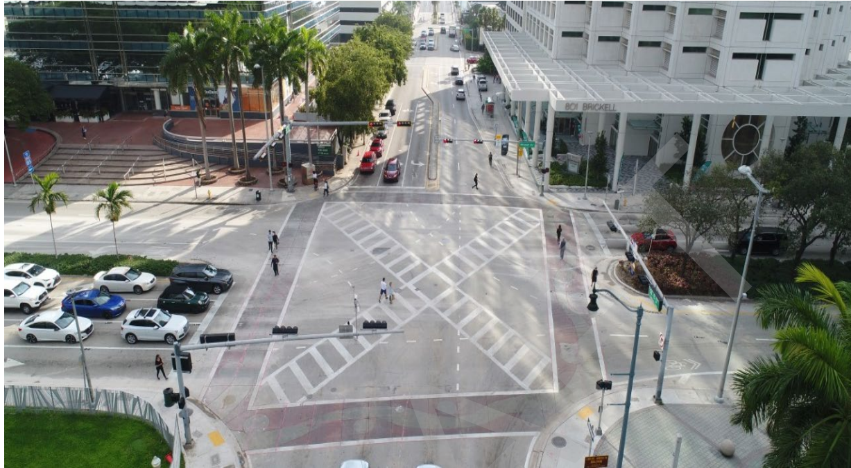
New Pedestrian Scramble Crosswalk at SE 8 St and Brickell Avenue
